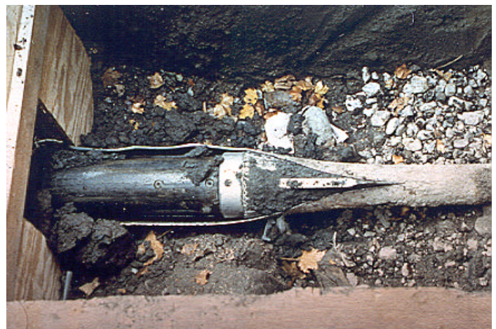
Photo of pipe being split by Con Edison
